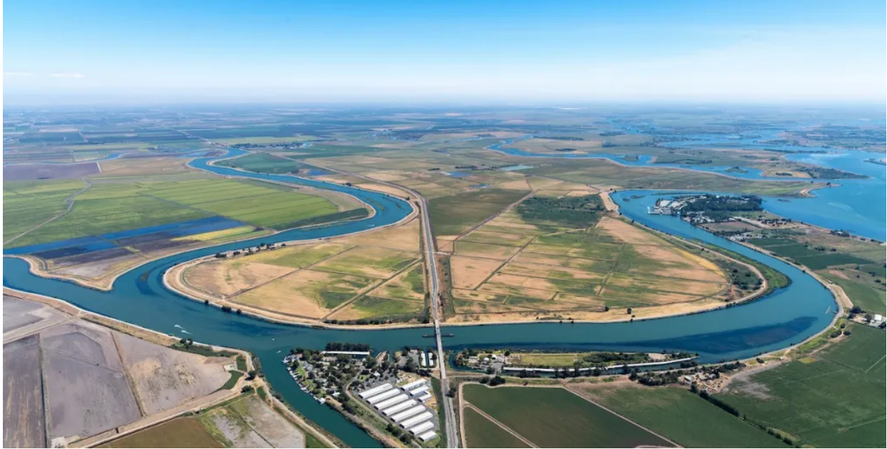
An aerial view of Highway 12 cutting through Bouldin island and crossing the South Mokelumne River in San Joaquin County, California. Photo by Ken James / DWR
